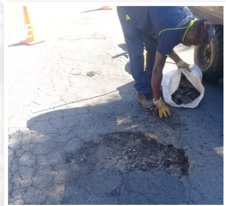
Repairs to numerous potholes on Braodacres Drive
