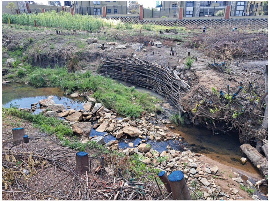
Repurposing the invasive trees, especially the black wattle, made for excellent natural barriers to curb erosion. You will note heavy scouring taking place at this section and critical areas were ascertained for installation.
