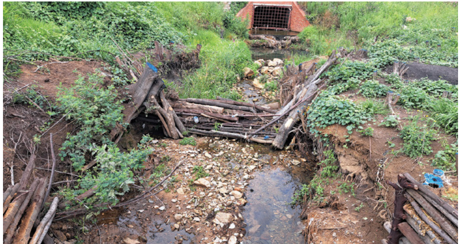
This is a naturally made dissipation and attenuation structure. It will slow down the water coming in from the top grate and allow for the deposition of silt and plant debris thereby allowing for other plants to take hold and lessen the deep channelling taking place.
