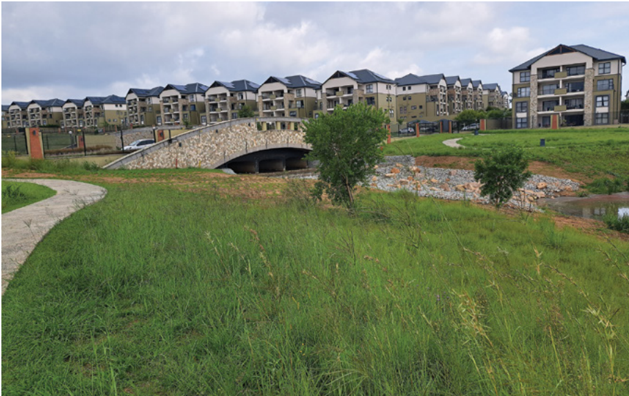
These two pictures depict the engineered solution which was required to prevent scouring under the bridge. This consisted of reinforcing the embankments with gabions including a fairly large dissipation structure just before the inlet of the dam. This will allow for any excess silt to be caught and cleaned prior to entering the dam.
